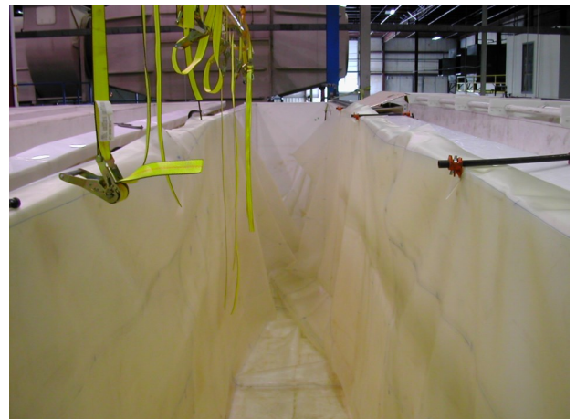
Spread liner across to opposite wall
