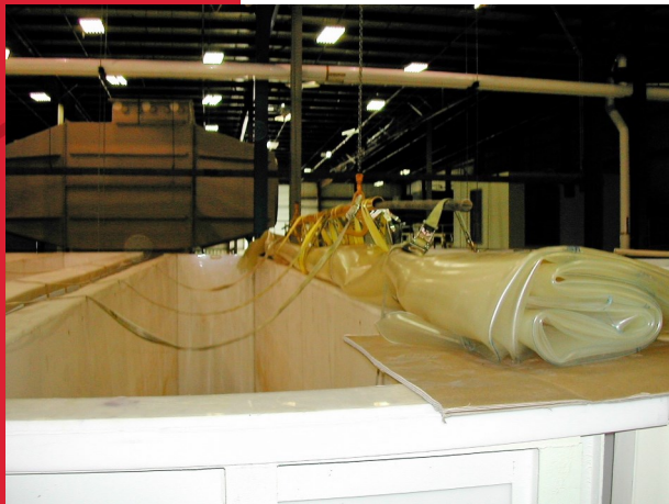
Unroll liner down tank sidewall
