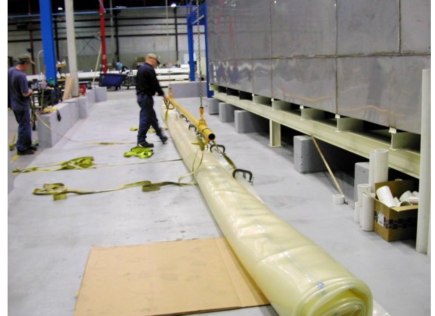
Secure liner for lifting to top of tank
